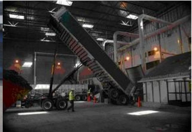
Biosolids are offloaded directly into receiving hoppers.
