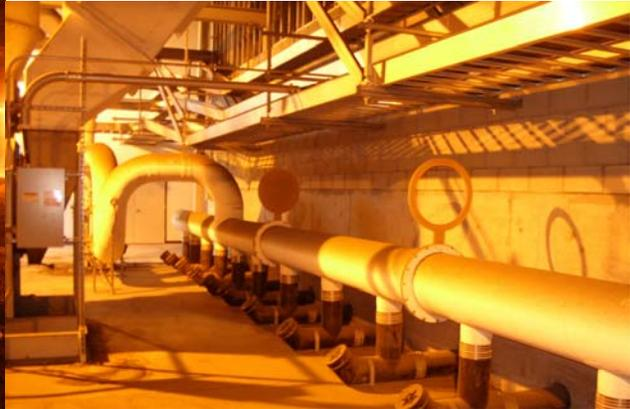
Fans, located in corridors within the building, pull air from the piles and exhaust it to a biofilter.
