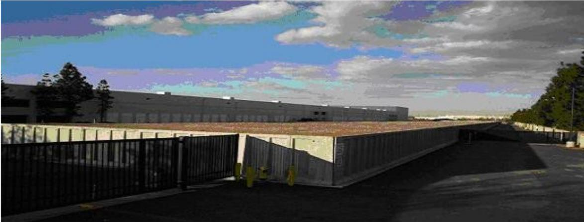
The biofilter contains over 50,000 cubic yards of chipped wood material piled onto a perforated floor. The facility exhaust air slowly travels through the 8-foot deep x 3-acre biofilter where odors and regulated compounds are removed.
