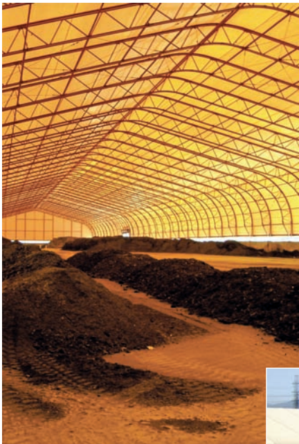
A fabric-covered building can hold nearly three months' production of compost (about 50,000 cubic yards). Storage space is often required during winter months, when sales are slower.
